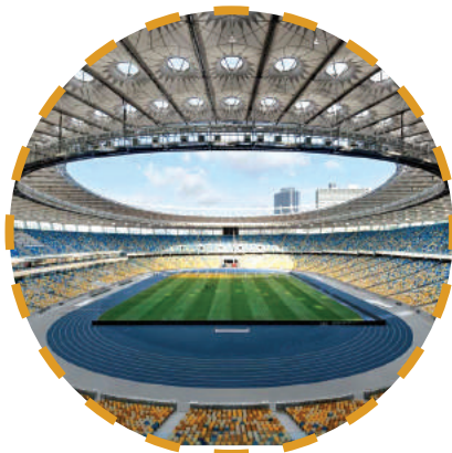
BROADCASTING INFRASTRUCTURE FOR SPORTS COMPLEX
